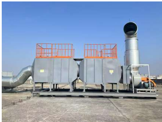
▲ After improvement (blower repair, fitting of shock-absorbing hoses and noise suppression piping)
